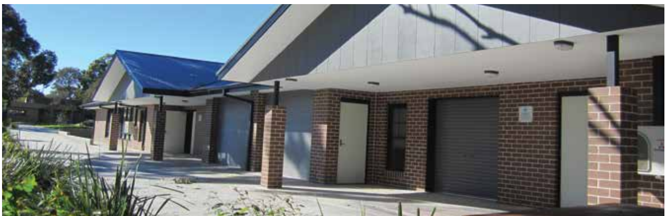
Completion of refurbishment. North West façade of building
